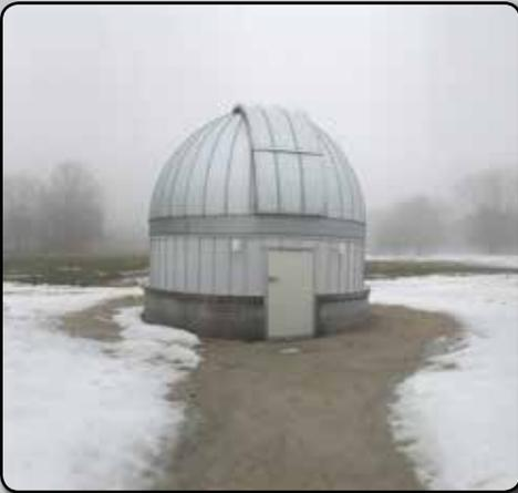
Installation of the Schoolyard Observatory dome was completed at the end of November 2016. The dome measures 5 meters (16 feet 5 inches) in diameter, and was manufactured by Ash Domes in Plainfield, IL.
