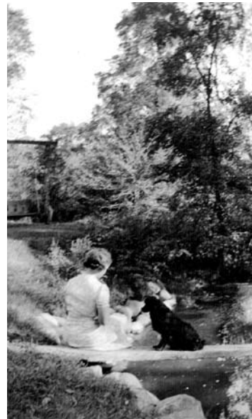
Margaret sitting on plank bridge over the Pike Creek around 1940. This bridge is at same location as our current bridge.
